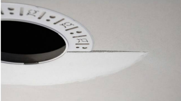
Partially finished mud ring, showing cross-section detail.
