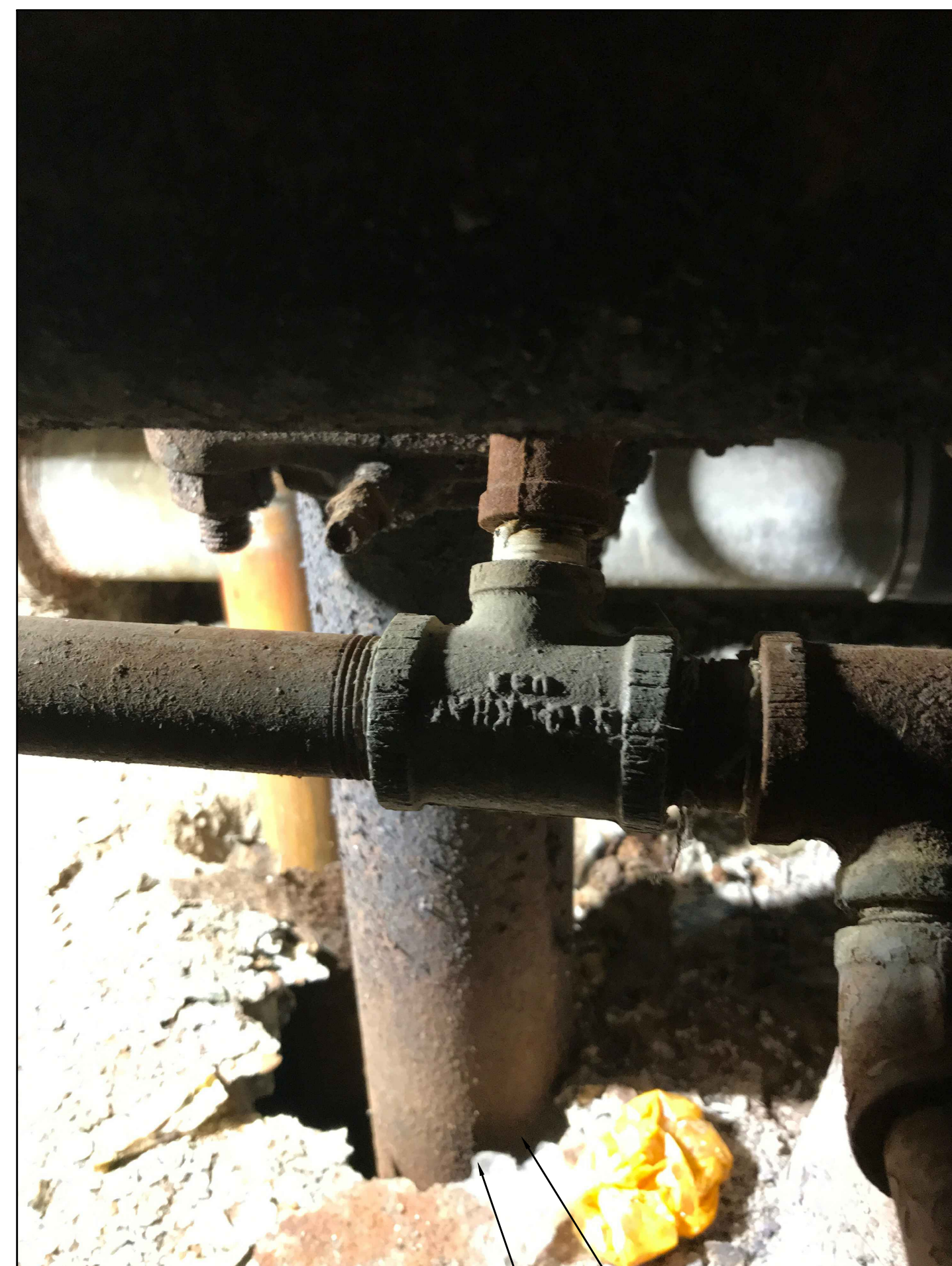
4" DCW PIPE PENETRATION OF CELL BLOCK PIPE CHASE FLOOR FROM TUNNEL
