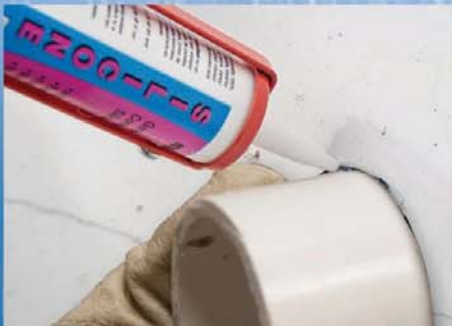
Seal wall opening with 100% silicone caulk.
