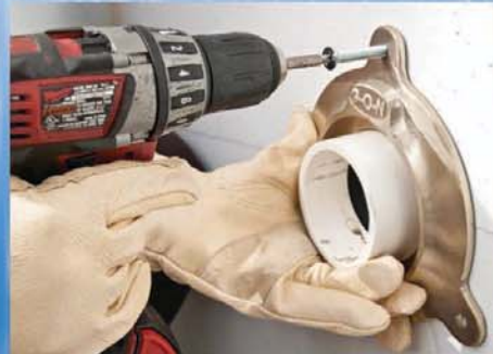
Install anti-theft escutcheon & secure with appropriate anchor.
