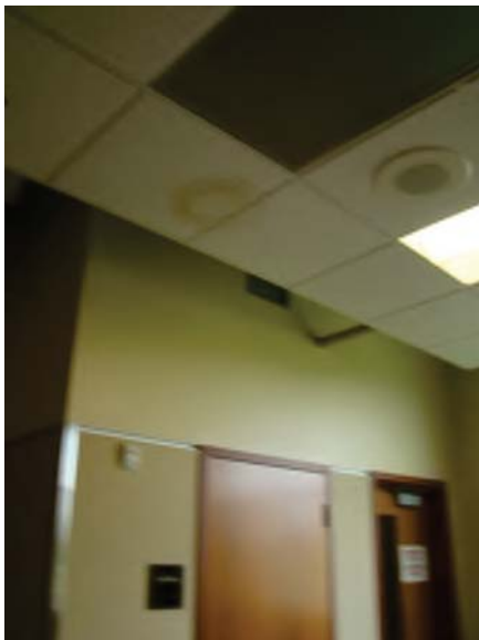
Figure B20.3 – Ceiling Tiles
