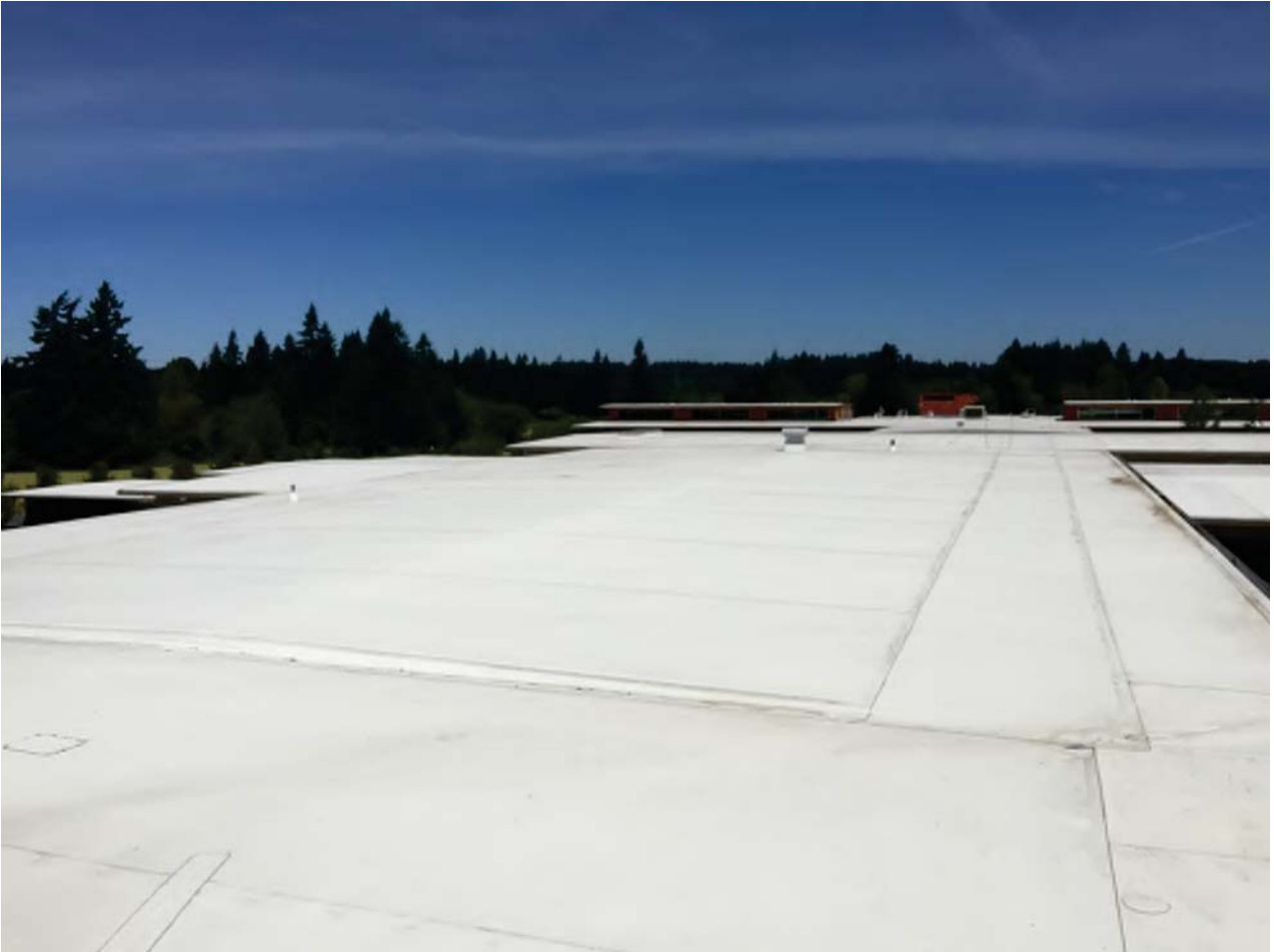
OPEN CLEAN ROOF WITH GOOD SLOPE
