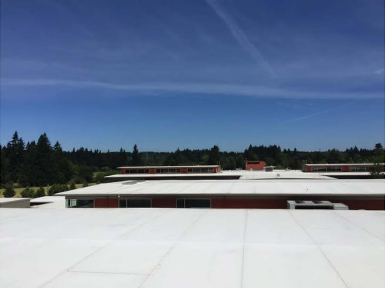
OPEN CLEAN ROOF WITH GOOD SLOPE
